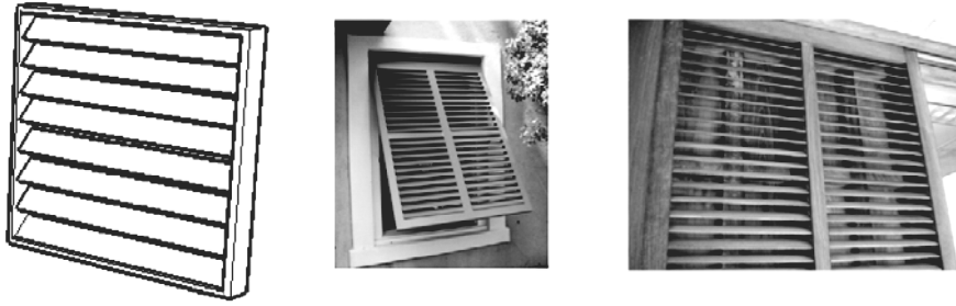
Figure 1 Examples of air intake louvers structure in buildings; source [2].
