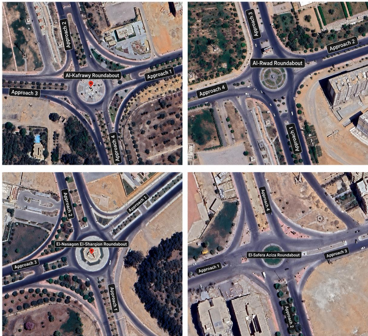
Figure 2 : Locations of the Selected Signalized Roundabouts in 10th of Ramadan City
