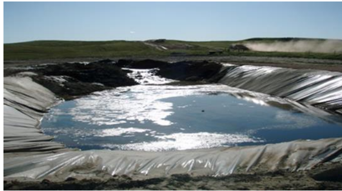
Figure 1: A lined pit used to store drilling fluids and rock scraps resulting from the drilling process. Insulating lining (plastic cover) helps prevent contaminants from seeping into the surrounding soil and groundwater
