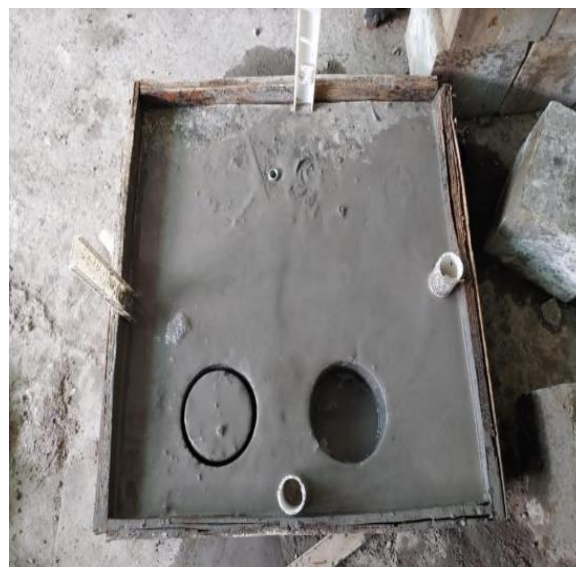
Figure No 4 Drilled Concrete Hole
